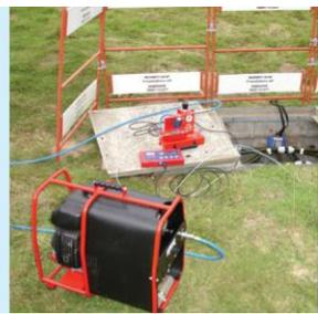
Developed from the 3A and now featuring an integral dispenser the 4A is the next generation in blown fibre technology. Incorporating an extremely efficient air delivery system the unit less airflow compared to the original 2A blowing heads. As a result this allows the units to blow to the same standard with considerably smaller air compressors, such as the petrol engine driven BT9A or 110/240V Electric Fibrevane, which both weigh under 25Kg.
