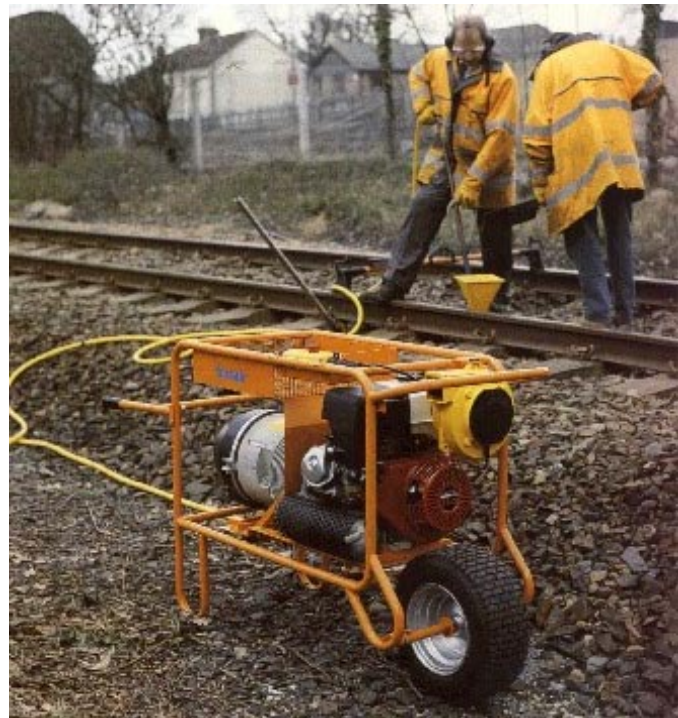
Railair unit being used for Stoneblowing
