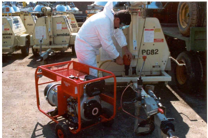
An engine driven unit being used to repair a mobile lighting tower.
