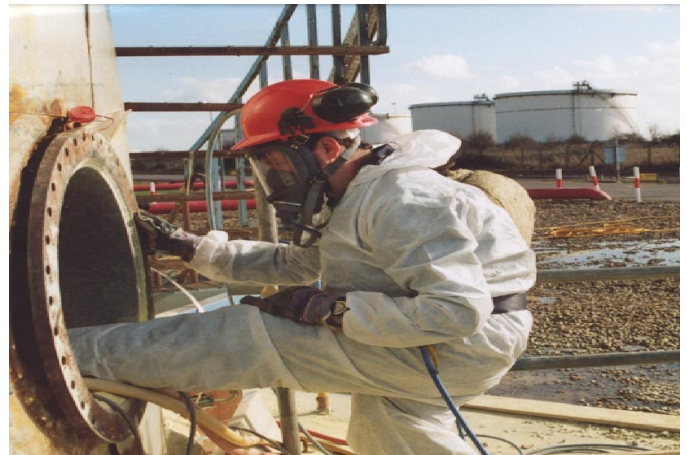
Operative wearing full breathing apparatus about to enter a maintenance hatch.
