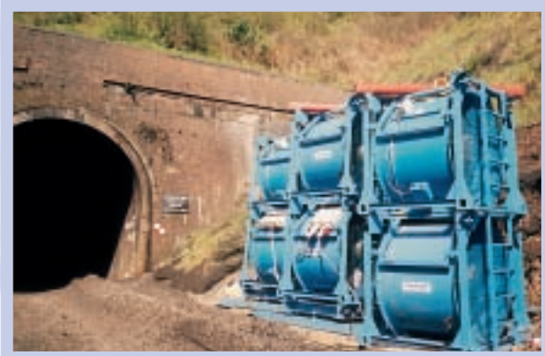
Ventilation Fans Deployed at Patchway Tunnel
